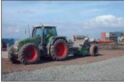
Rolling dynamic compaction of base layer
