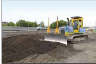
Blading out site-won material before in-situ stabilisation
