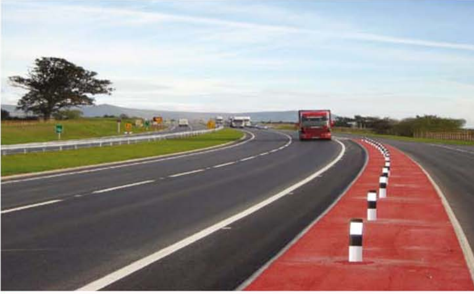
A66, Temple Sowerby, the finished bypass in use
