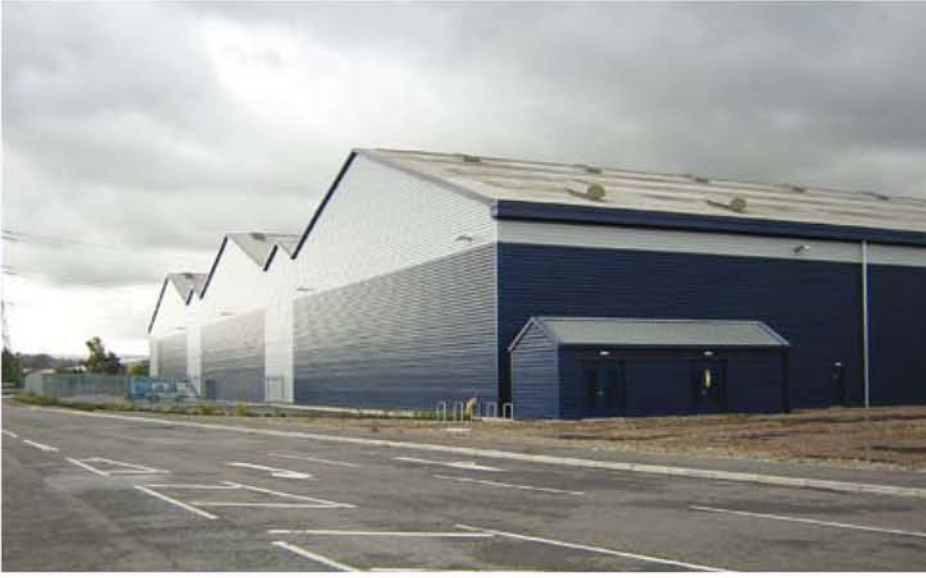
The refurbished building ready for use as warehouse/distribution centre
