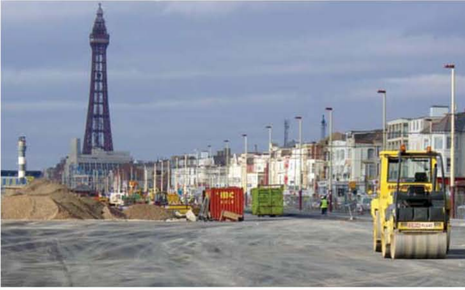
Rolling out the temporary blacktop over the stabilised bulk fill
