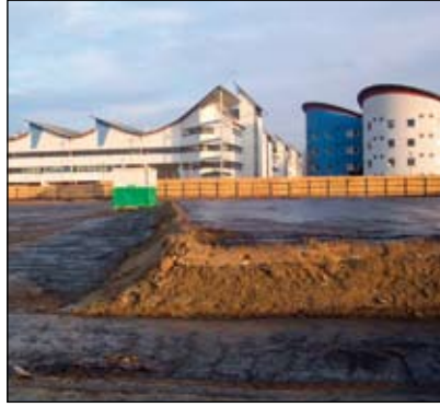
The completed stabilised platform after application of bitumen tack coat
