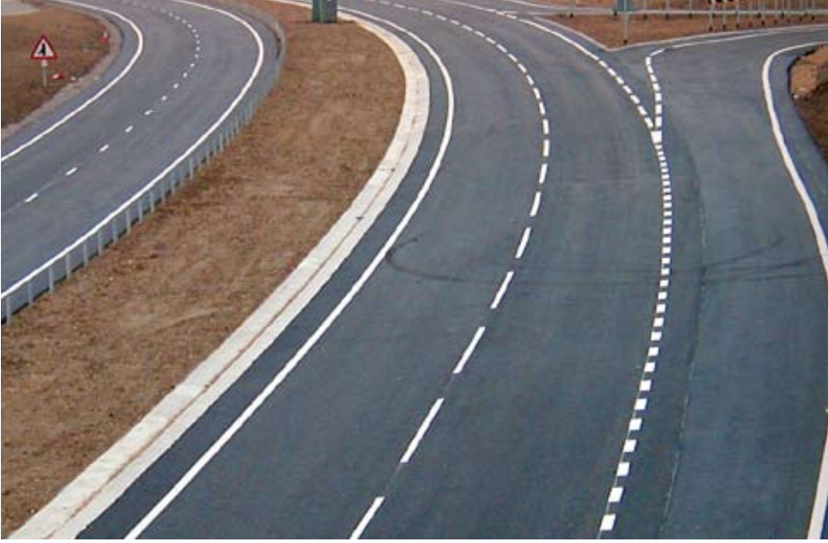
The A6 north of Bedford built on engineered capping material
