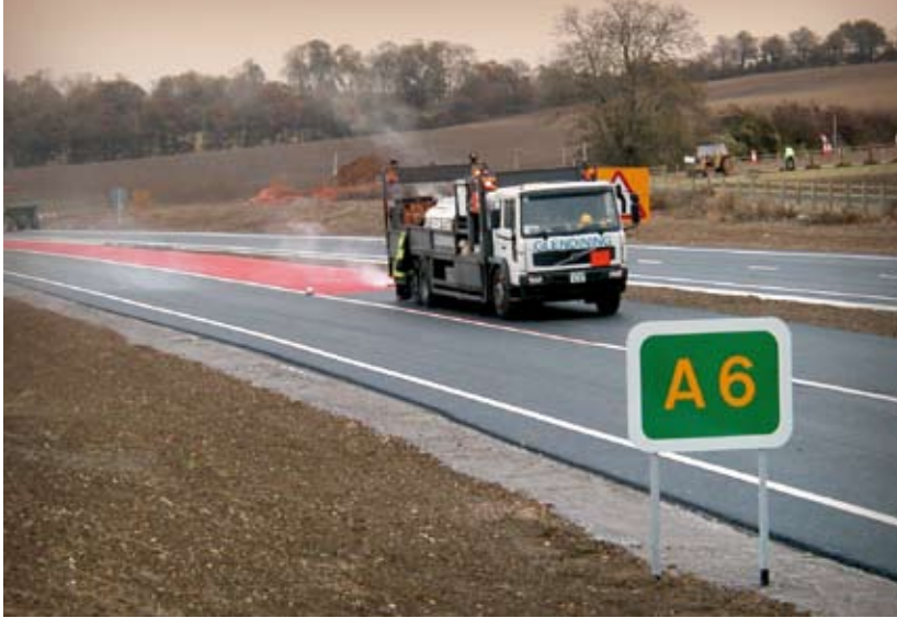
Work in progress on the A6
