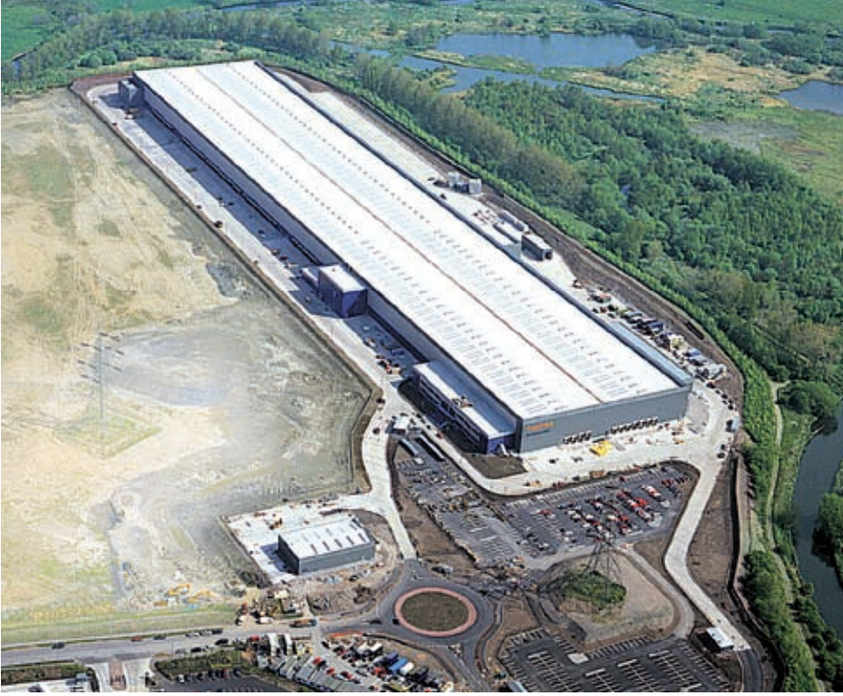
This large distribution centre was successfully completed to a tight programme (The area to the left is another plot yet to be treated)
