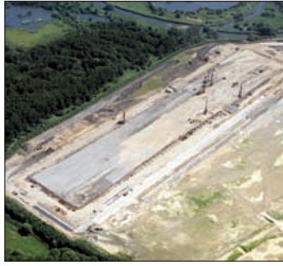
Arial view of the site showing stabilisation in progress
