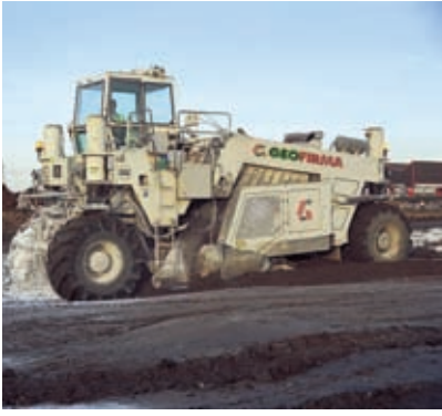
Incorporating the cement into the pulverised fuel ash
